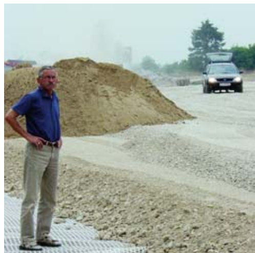
Construction of the drilling pad: 1) Grading 2) Plastic liner 3) Approx. 1/2 m course gravel 4) Approx. 25 cm fine gravel and approx. 10 cm asphalt to come.
