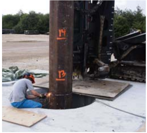
Cutting the conductor pipe in the cellar. The well will be drilled through this pipe.
