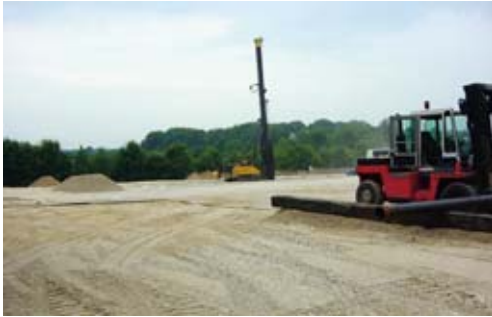
Location viewed from the casing area.
